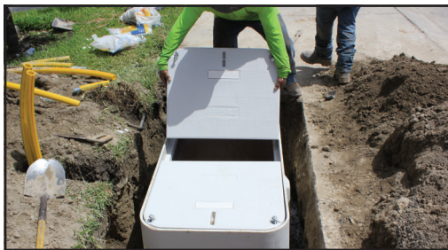
Optional split lid covers facilitate lid removal, access, and technician safety
