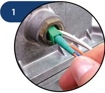
1 Feed connectors through node entry port
