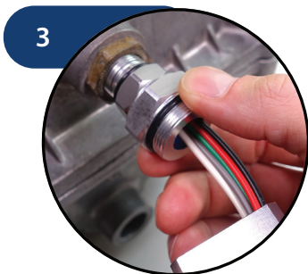
3 Thread coupling fitting a full turn into node
