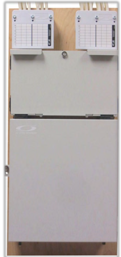
Microduct Manifold with Slack Storage & FSB
