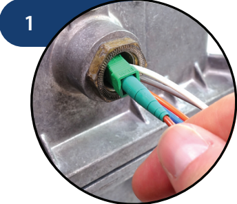
1 Feed connectors through node entry port
