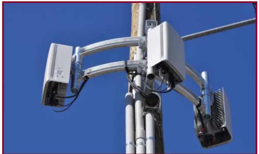
97-5GWDMTHGN1-A installation with (3) customer-supplied 5G radios
