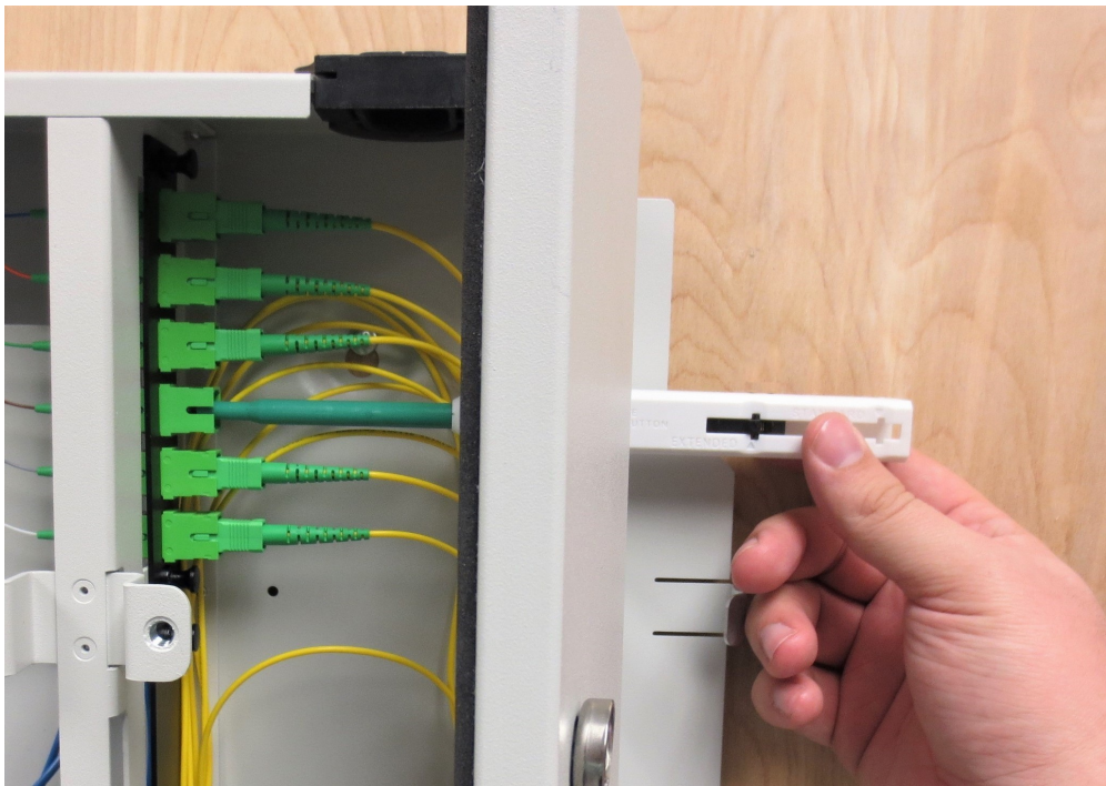
Optical Port Cleaning Tool use with FDE
